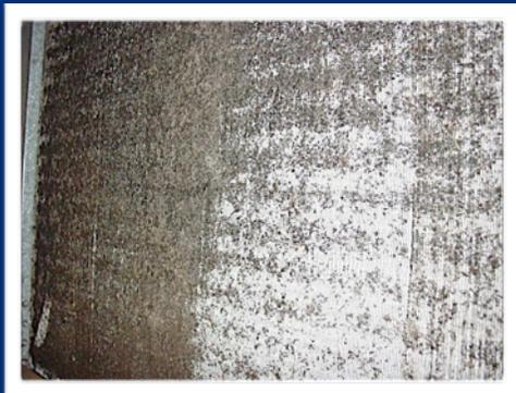
*Dirt Accumulation on Coils*
